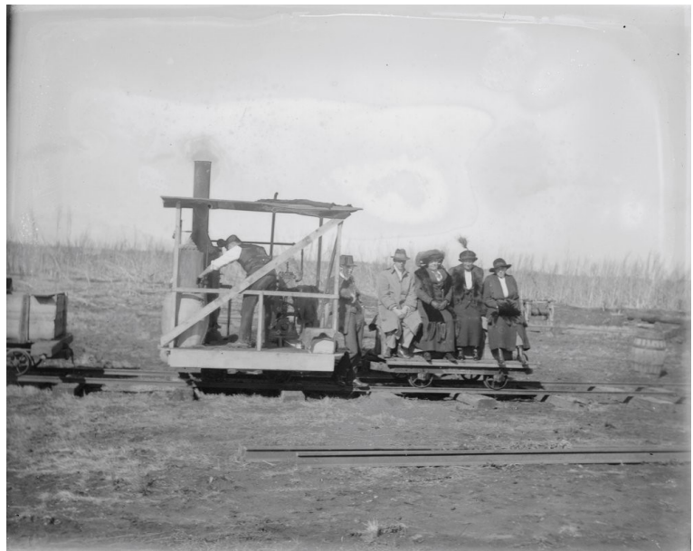
This is the Tangye engine referred to, used to haul machinery, goods and in this case important visitors taken on May 21, 1914, the day the Dredge was officially started.
